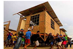
Transitional Shelter (2011) 01_Α-Γ | 02_Ε | 03_Α | 04_ΣΤ | 05_Β | 06_ΣΤ | 07_Β | 08_ΣΤ | 09_Β | 10_Ε
